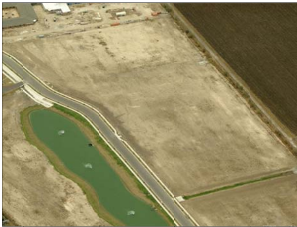
Figure 1: Pre-Construction Birds Eye View
